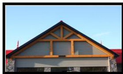
30' x 12' Timber Truss - Wasaga Beach, ON
